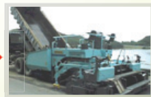
Asphalt pavement material, etc.
